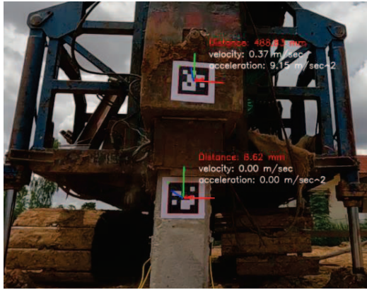
Fig. 3 The ARUCO target installation during testing
