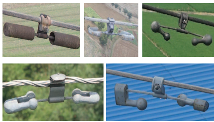
Fig. 1. Different shapes of vibration dampers.
